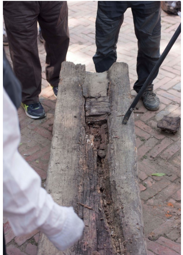
Figure 6: Inspection of One of the four main central posts, earlier repair had sealed the damage with wood dust, glued in place with wood chunks
